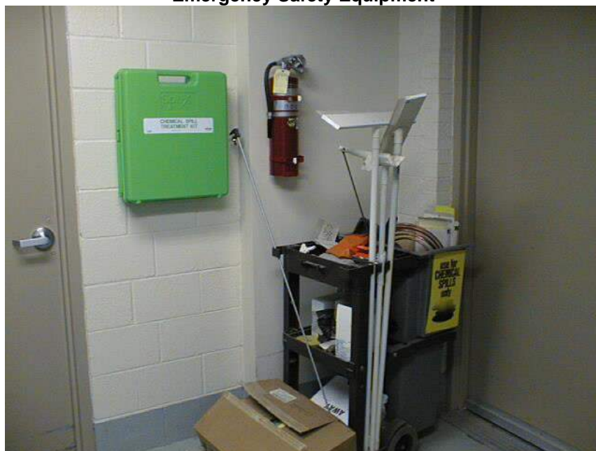
Spill kit, fire extinguisher and spill cart inside cleanroom
